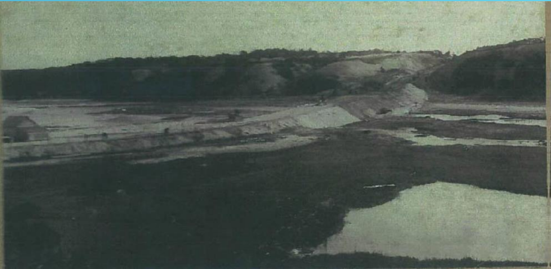
Historic photo of earthen fill placement at Orleans Road (Route 28) over Muddy Creek, facing south toward Chatham circa 1900
